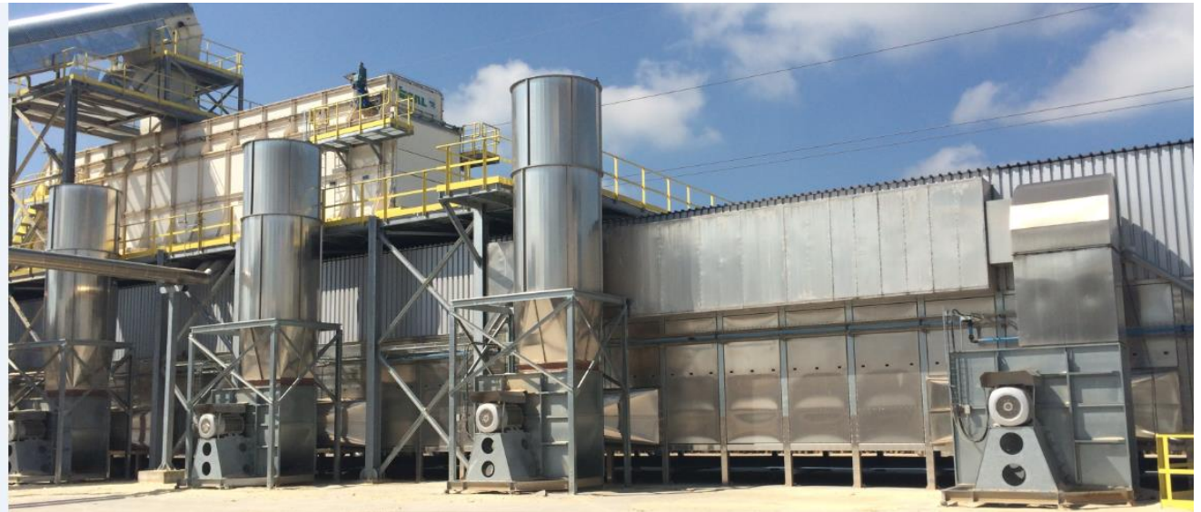
Fig. 11 belt dryer on which Stela has conducted research and made modifications within the scope of the project
