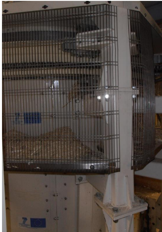
Fig.9 another view of the cone-shaped rotary chute
