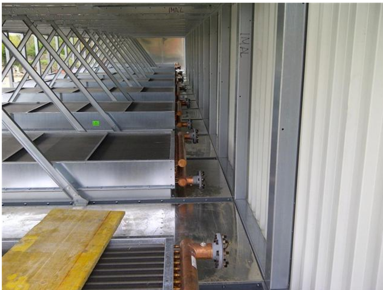
Figure 8 – installed heat exchangers in the exhaust air area
