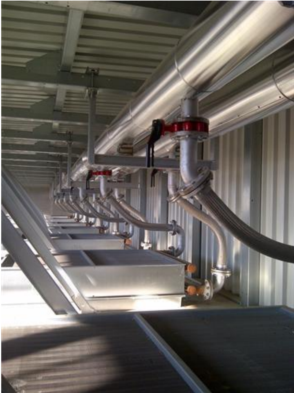
Figure 10 – additional installed heat exchangers with piping
