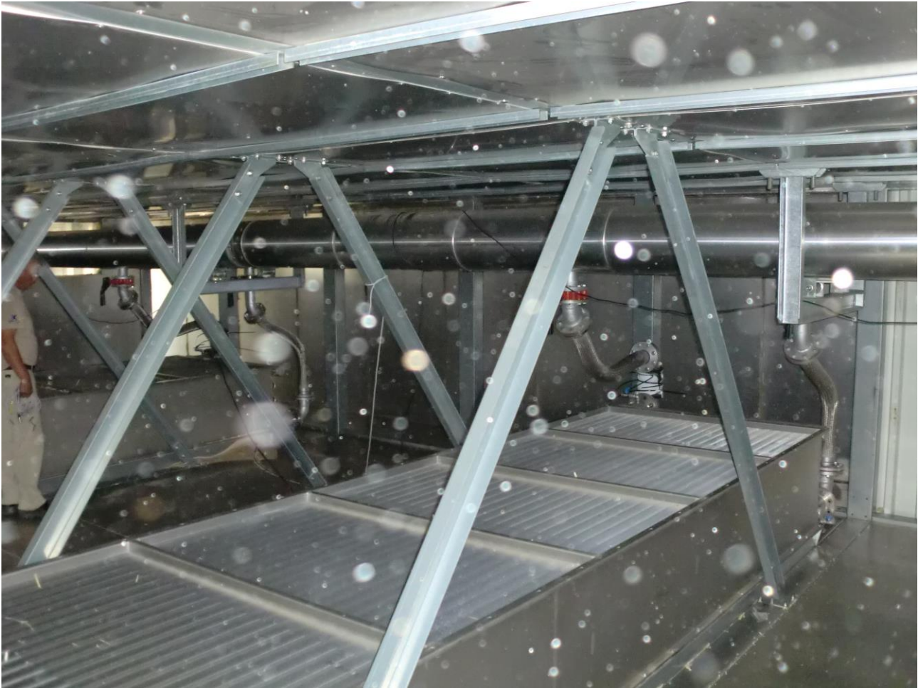
Figure 9 – installed heat exchangers in the circulation air area
