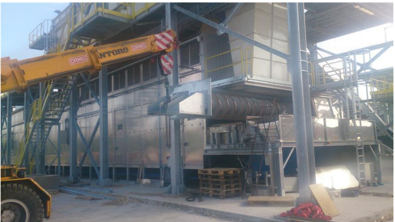
Figure 5: modification works on the product distribution screws and screw-through
